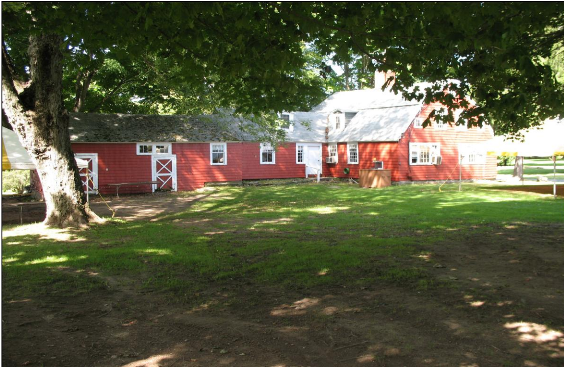
Picture 1. Toll House (Building #82) This structure is DEP's highest priority for preservation and re-use.
